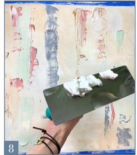
**4 | APPLY** an even, thin layer of the 3a mixture from Step 3 on the whole surface area using the medium plaster trowel (*Photo 6*).
