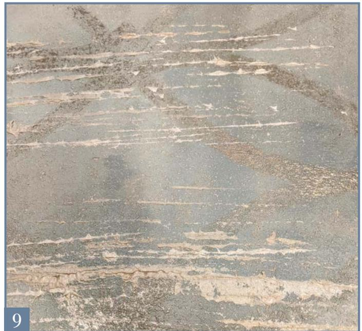
**5 | SAND** the peaks with 220 grit sandpaper (using a sander for large areas) to reveal the original untinted weathered granite (*Photo 6*).
